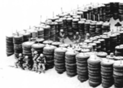
Figure 24. Tire Revetment Walls.
